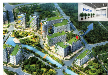
Dongguan Haihong : R&D center in South China
